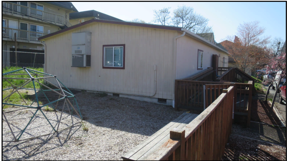
North facing wood framed 1-story modular building, constructed in approximately 1996.
