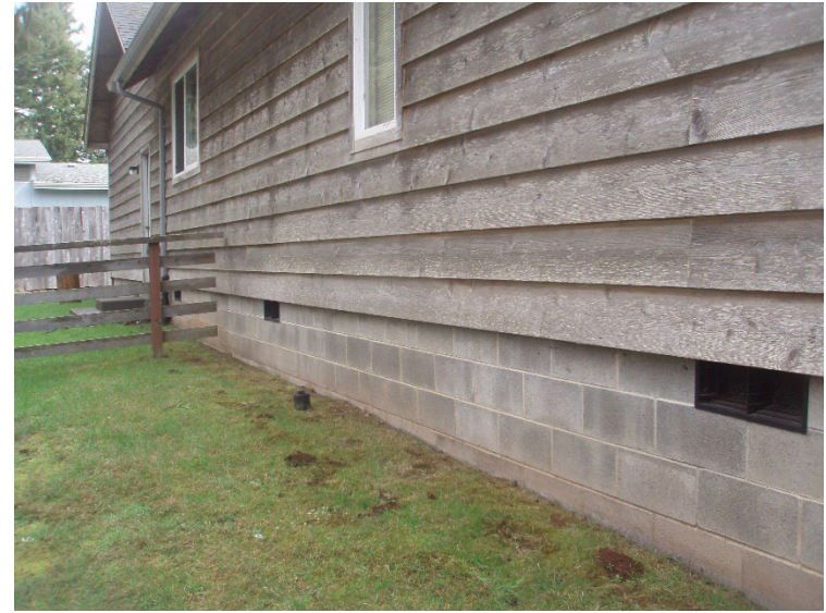
Masonry block foundation on north side of rental house – view east.
