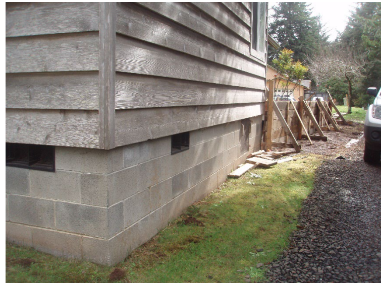
Masonry block foundation on west side of rental house – view south.
