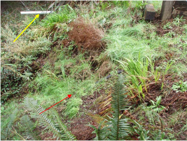
Drainpipes (center and upper left) discharging to slope. Vertical post in upper right is on east boundary of subject property.
