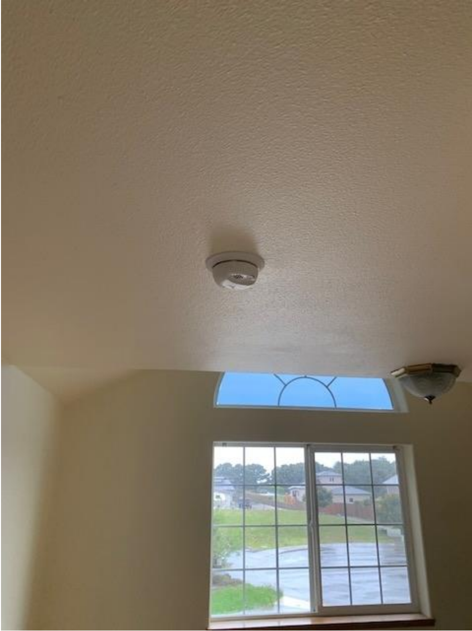
Smoke alarm in master bedroom
